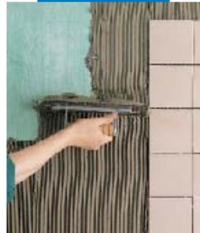
Laying on gypsum treated with Primer G
