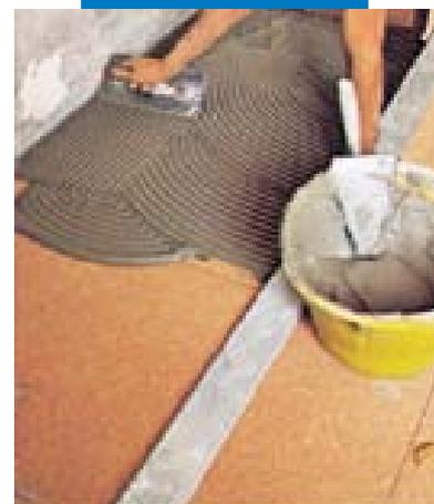
Laying on an insulating layer of cork in a tunnel prefabricated building
