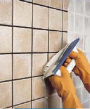
Single fired tile wall grouting with a trowel
