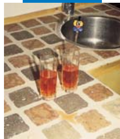
An example of a bonded and grouted kitchen bench
