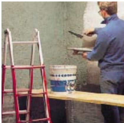
Adhesive render admixed with PLANICRETE SP
