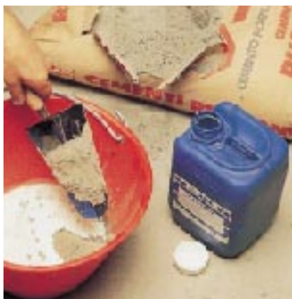
Mixing cement mortar with PLANICRETE SP
