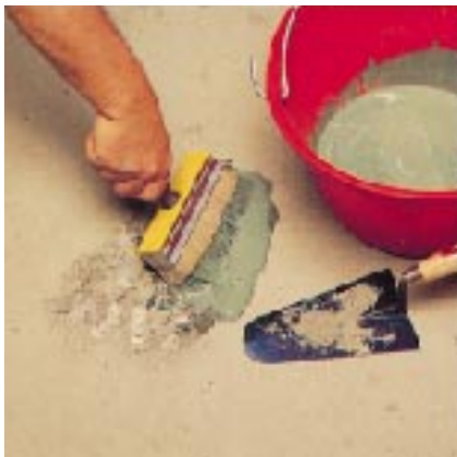
Floor patching: application of slurry
