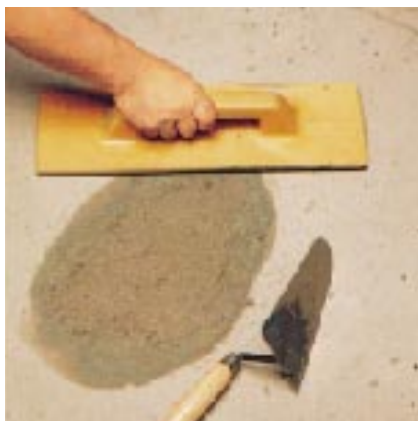
Floor patching: final smoothing
