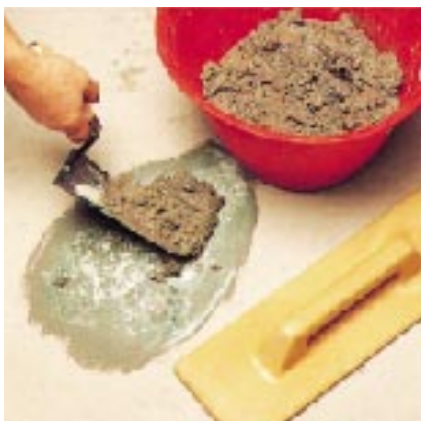
Floor patching: application of mortar
