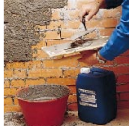
Adhesive shotcrete modified with PLANICRETE
