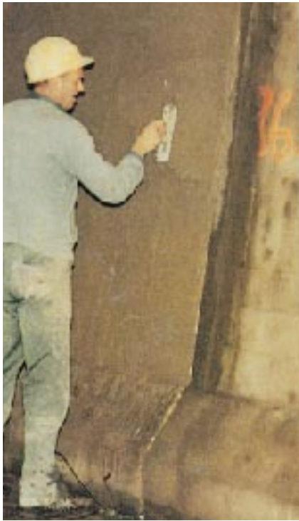
Cement plaster with PLANICRETE. Ville Marie motorway tunnel, Montreal, Canada
