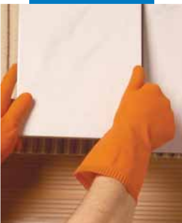
Installation of ceramic tiles on a wall
