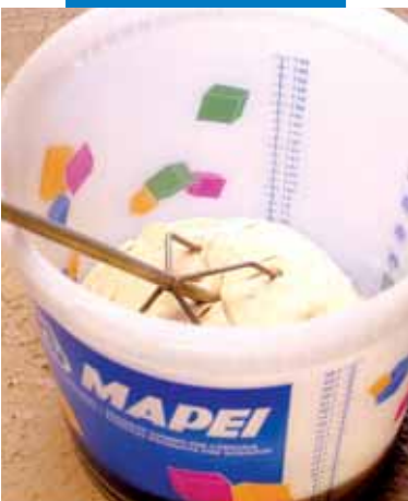
Mapeset mix made with mechanical stirrer
