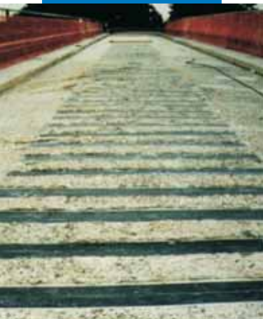
A bridge-deck reinforced with Carboplate
