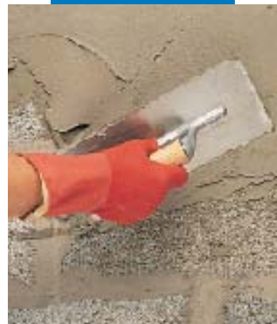
Application of Idrosilex Pronto by trowel
