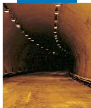
Application of white Idrosilex Pronto by spray gun in highway tunnel
