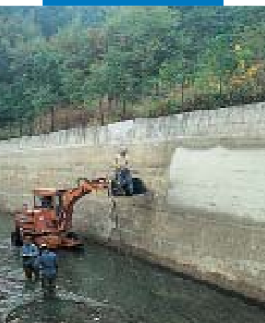
Application of Idrosilex Pronto by spray gun in hydroelectric canal
