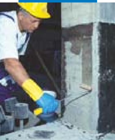
Applying a first coat of Mapewrap Primer 1
