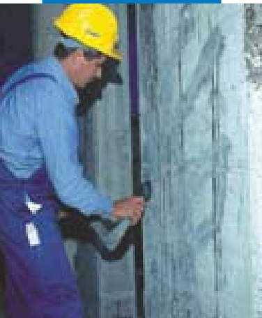
Preparing the substrate
