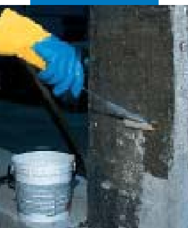
Applying a second coat of Mapewrap Primer 1
