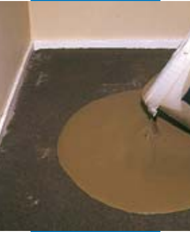
Applying the Novoplan 21 paste on the substrate
