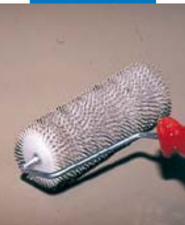
Using a spiked roller over a fresh coat of Novoplan 21
